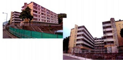
Existing Building 樓宇現貌
